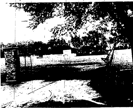
A FAMILIAR LANDMARK to sports fans in the Wayne area was ruined Monday following a Wayne-Wakefield baseball game. One of the brick pillars at the south gate of the ballpark crumbled when it was accidentally backed into by a Wakefield woman.
